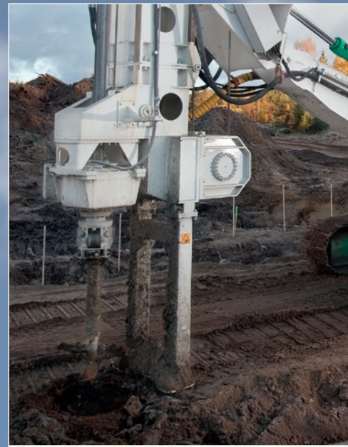
Dry Deep Mixing
