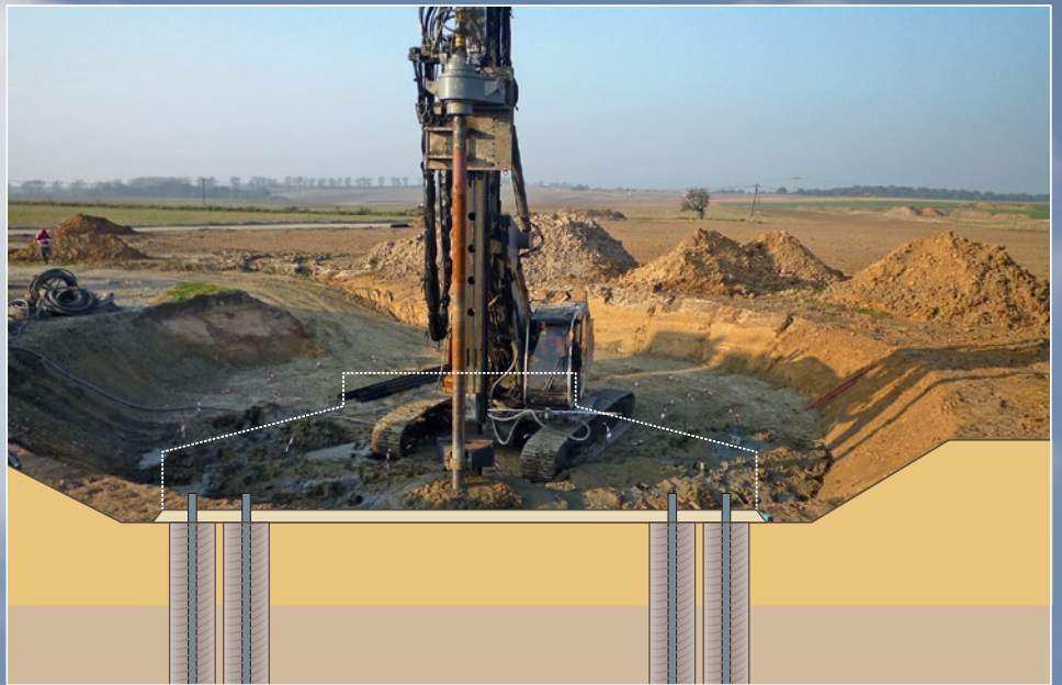
Wet Deep Mixing
