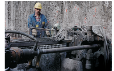
Installation of Soilfrac® borings
