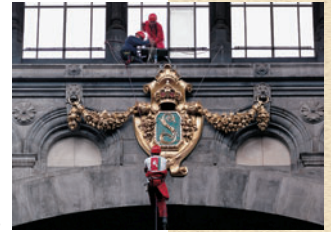
Installation of a crack thickness measuring device
