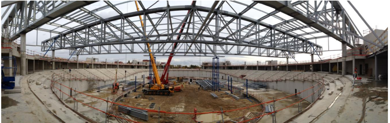
FIGURE 6: STRUCTURE EN TREILLIS - VELODROME DE SAINT QUENTIN
