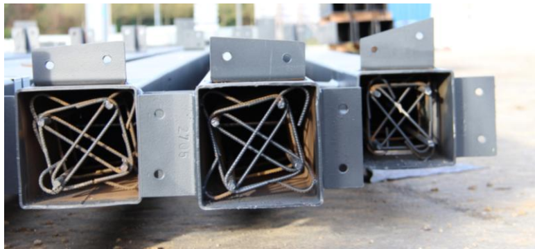
FIGURE 10: POTEAUX MIXTE ACIER/BETON
