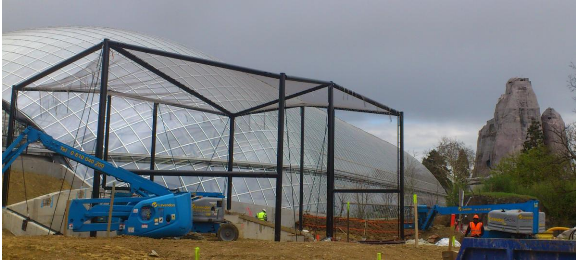
FIGURE 7: STRUCTURE TUBULAIRE - ZOO DE VINCENNES
