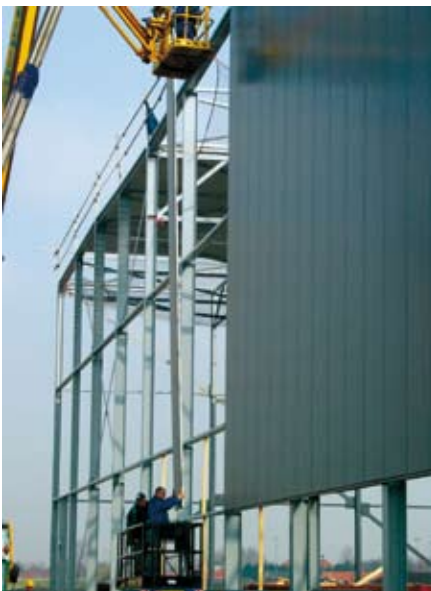
Figure 5.6 Panneaux-sandwich
